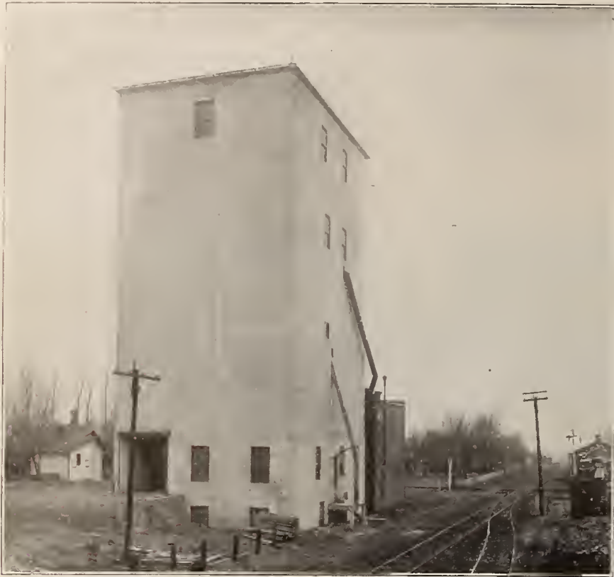
Concrete Fireproof Grain Elevator built for the Crabbs-Reynolds-Taylor Co. at Wingate, Ind. Capacity 60,000 Bushels.
